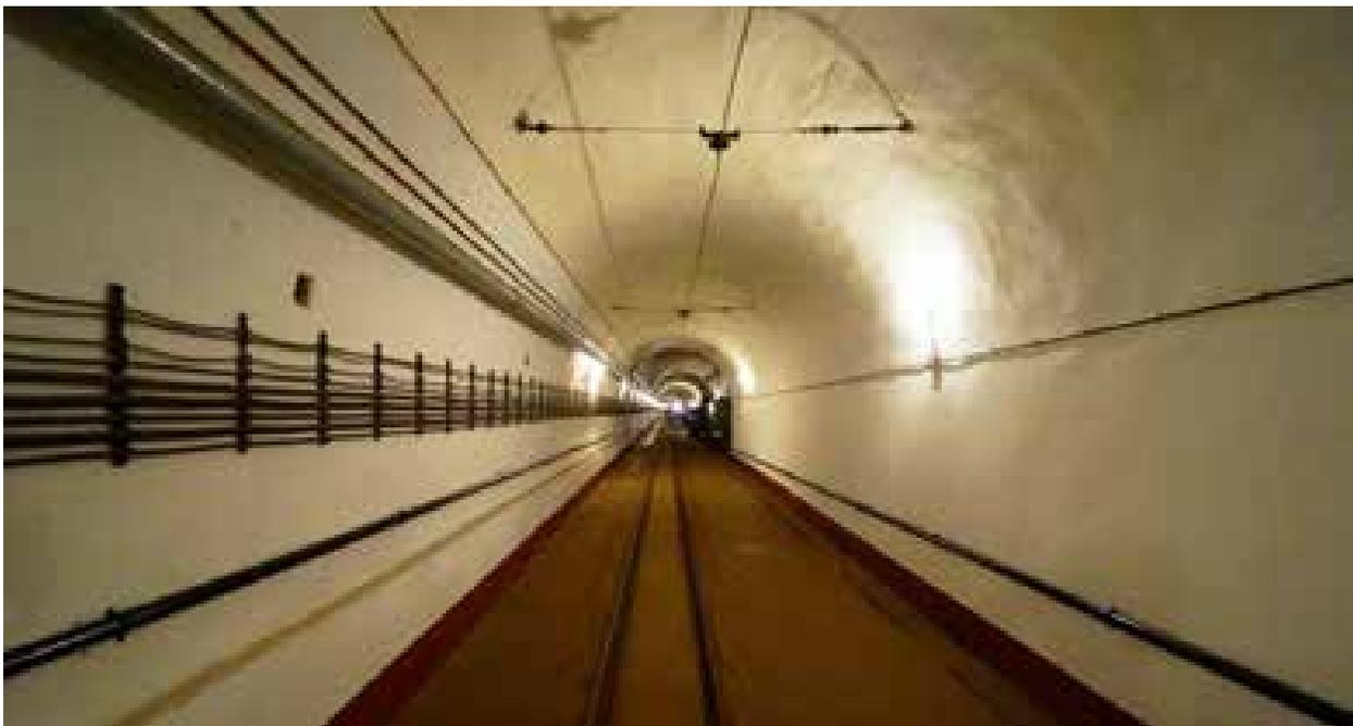
Fig. 9. Paul Painleve & C.O.R.F., the lifeblood of the fort, telephone and electrical lines run the length of the tunnel, *Ouvrage Hackenberg*, Vekring, France, 1929-1932.
