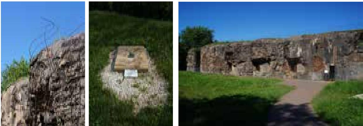
Fig. 12-14. Paul Painleve & C.O.R.F., views of Block 8's façade and adjacent American memorial with steel reinforcement exposed from the Allied assault, Ouvrage Hackenberg, Vekring, France, 1929-1932.
